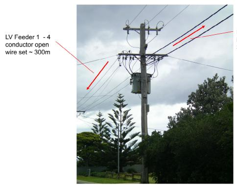
LV Feeder 2 - 2 x aerial bundled conductors ~ 300m
